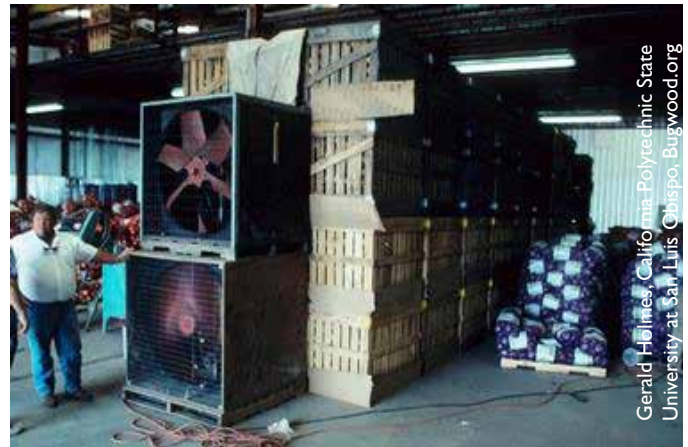
Fans inside cooling rooms are used to cool produce quickly to reduce damage caused by respiring fruit.
